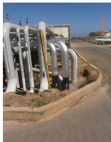
KERO JET A-1 PIPING MODIFICATION TANKAGE AREA - PETRON BATAAN REFINERY
